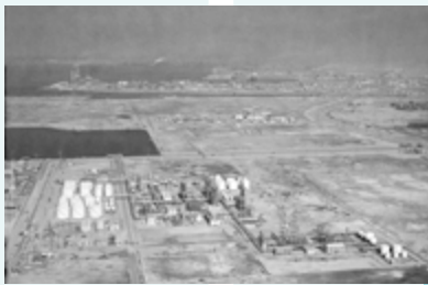
Nissan Petrochemicals Chiba Plant (1968)
